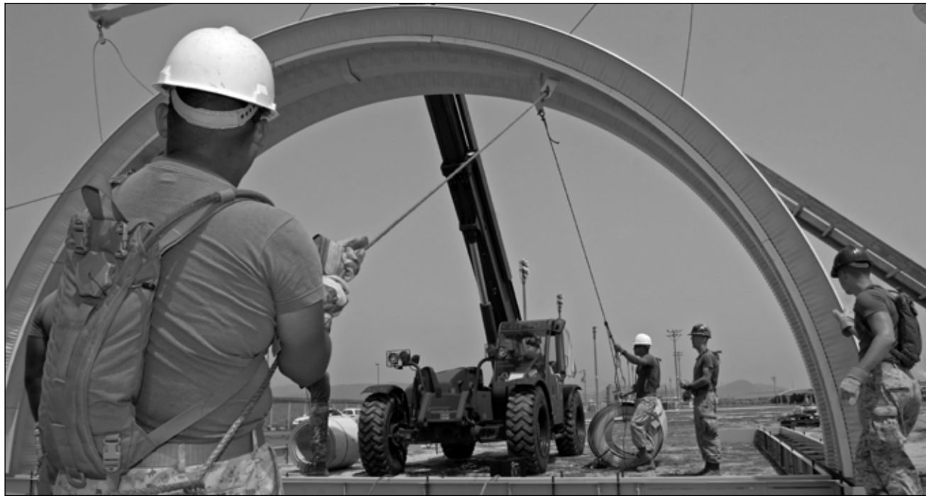
With the assistance of a Millennia Military Vehicle, combat engineers from Marine Wing Support Squadron 171 raise a steel structure into its foundation at Penny Lake May 8. For 12 days the Marines trained with the Ultimate Building Machine, a mobile piece of manufacturing equipment capable of quickly producing buildings without the need of nuts, bolts or trusses. Photo by Lance Cpl. Noah S. Leffler
