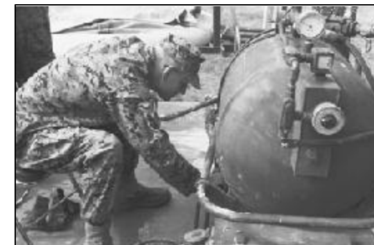
Lance Cpl. Shawn Gardner, Marine Wing Support Squadron 171, adjusts the valves on a water pump during the field mess exercise.
