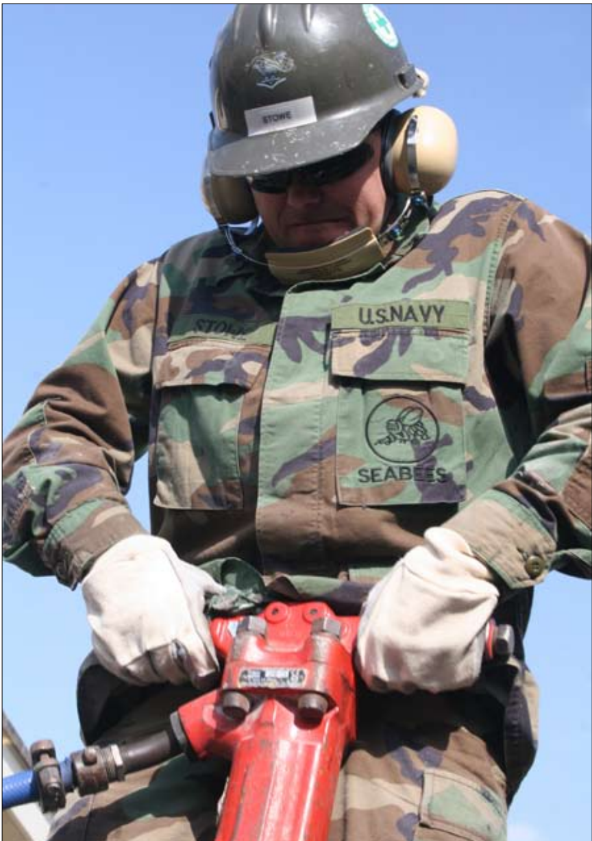
Builder 3rd Class Michael R. Stowe, one of the 22 Seabees serving here with station facilities, breaks up concrete behind the commissary to make way for a new construction project. Stowe and his fellow Seabees take special pride in wearing the Seabee patch and being part of the Seabees’ rich history and tradition.
