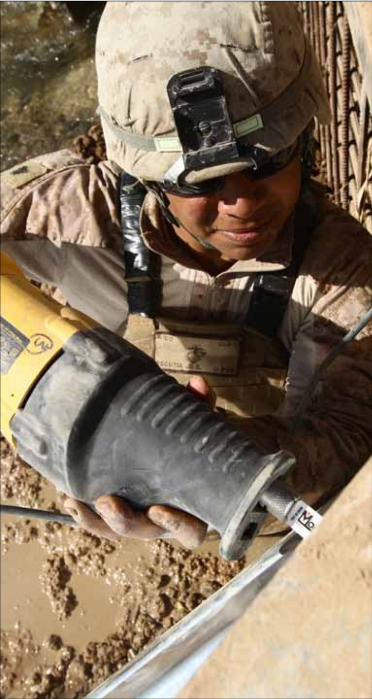
LANCE CPL. ALFRED V. LOPEZ U.S. Marine Cpl. Samuel Escutia Jr., a combat engineer with Alpha Company, Combat Logistics Battalion 1 and 21-year-old native of Reedley, Calif., cuts through a wing-wall here, Nov. 12. Marines of Alpha Co. are currently repairing the support structure on a bridge located at a major intersection that connects Marjah and Nawa districts. The bridge receives heavy foot and vehicle traffic due to the local bazaar, as well as Afghan and coalition military convoys.
