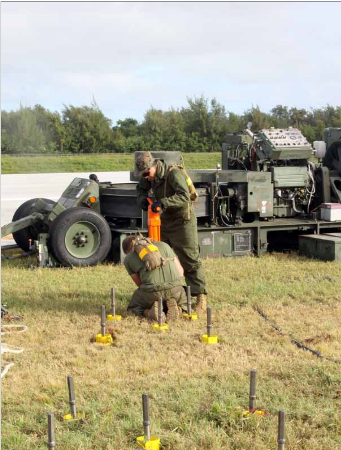
Marines use a jackhammer to drive anchors in place for an M-31 Marine Corps Expeditionary Arresting Gear System at Tinian's West Field Dec. 2 during Exercise Forager Fury 2012. The MCEAGS' two trailers are set on opposite side of the airstrip 250 feet apart and will be able to allow F/A-18 Hornet aircraft to perform arrested landings every 3-5 minutes during the exercise. The Marines are Expeditionary Airfield System Technicians with Marine Wing Support Squadron 171.
