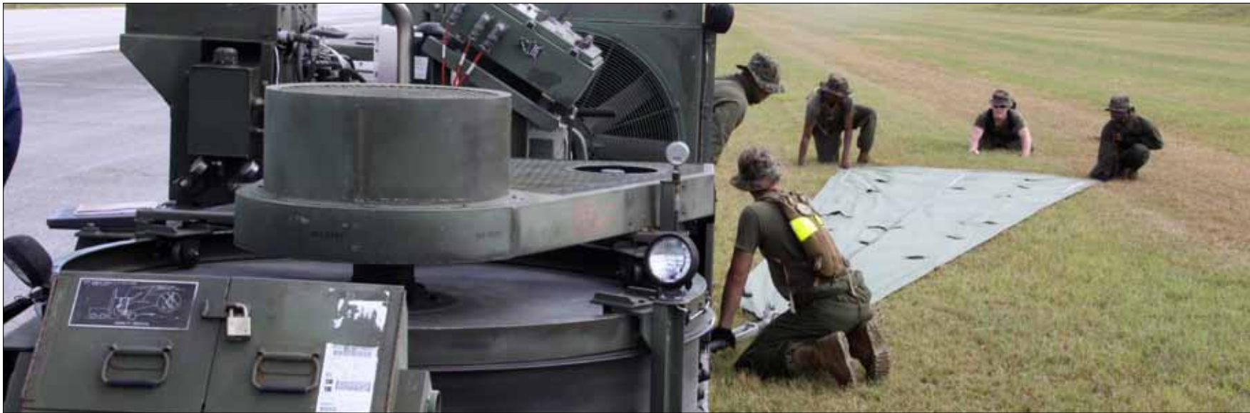
Marines lay a stick placement template next to an M-31 Marine Corps Expeditionary Arresting Gear System at Tinian's West Field Dec. 2 during Exercise Forager Fury 2012. The template assists the Marines in marking the ground where they will drive in anchors to keep the trailer in place.
