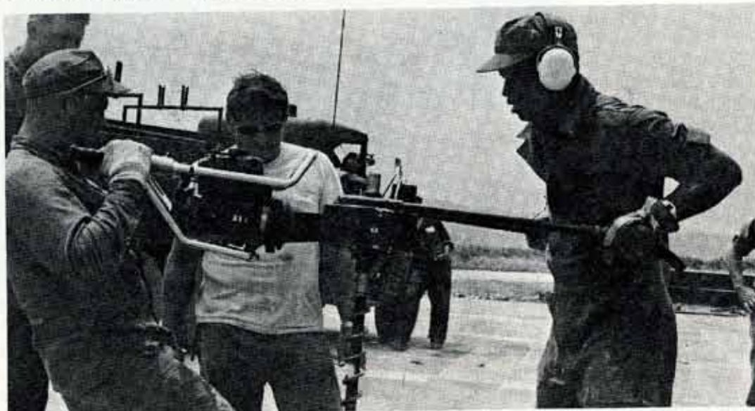
EARTH ANCHOR - Sgt. Steve D. Metroff (left) and LCpl. Rodney L. Johnson prepare to drill a hole for an earth anchor. This is just one of the many processes involved in the construction of a vertical landing pad for AV-8A Harriers.
