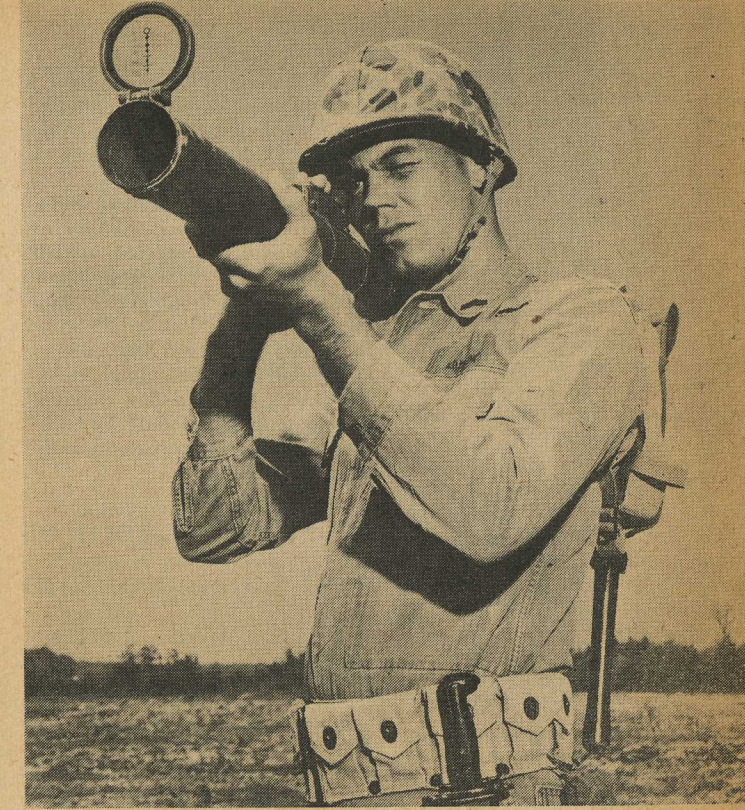
"SIGHTING IN" -- Among the experimental weapons currently undergoing test is this light anti-tank weapon (LAW), which resembles a sawed-off 3.5 rocket launcher (bazooka).
