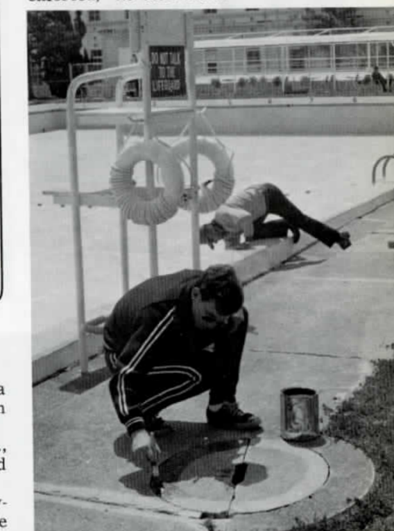
LCPL. KENNETH K. GILLIS REPAINTS SAFETY MARKINGS ON THE DECK OF THE MAINSIDE SWIMMING POOL, WHILE SSGT. LAWRENCE P. TRACKEY, NCOIC OF THE SPECIAL SERVICES POOLS, INSPECTS THE WALLS. WORK IS WELL UNDERWAY TO GET THE POOLS IN SHAPE FOR THE UPCOMING SWIMMING SEASON.
