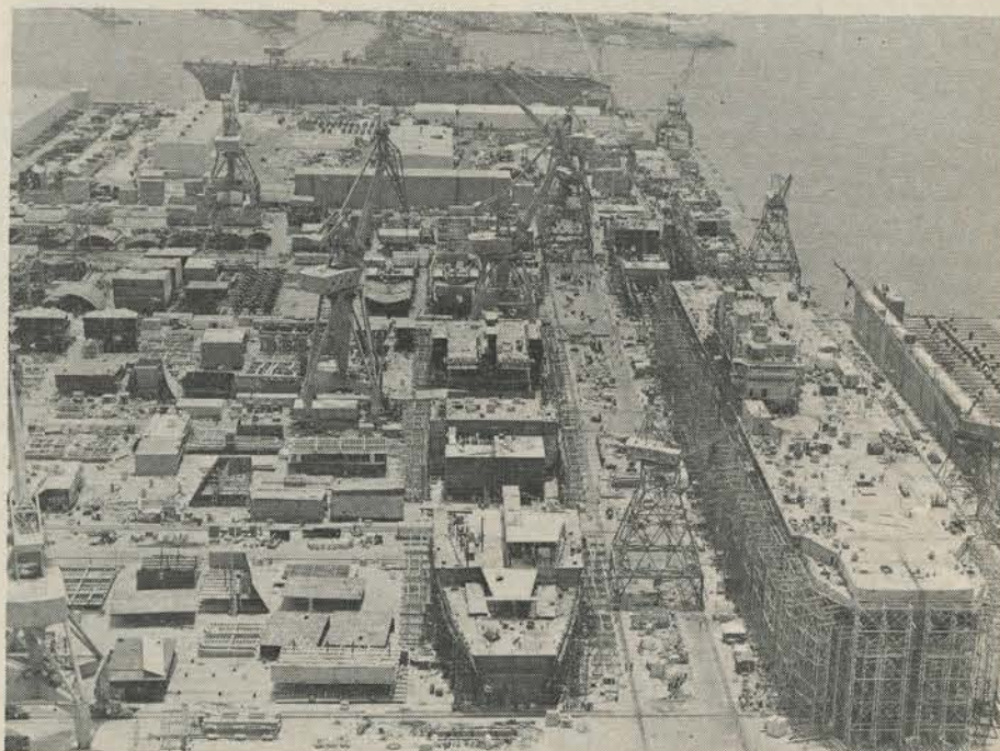
THE USS SAIPAN, LHA-2, SITS AT THE RIGHT SURROUNDED BY HIGH SCAFFOLDING AT THE INGALLS SHIPBUILDING YARD IN PASCAGOULA, MISS., WHILE WORKMEN MAKE HER READY FOR LAUNCHING. THE SAIPAN WILL JOIN HER SISTER SHIP, THE USS TARAWA, LHA-1, VISIBLE IN THE BACKGROUND, FOR COMPLETION. THE USS BELLEAU WOOD, THIRD IN THE SERIES OF GENERAL PURPOSE AMPHIBIOUS ASSAULT SHIPS, SITS ON THE IMMEDIATE LEFT OF THE SAIPAN.
