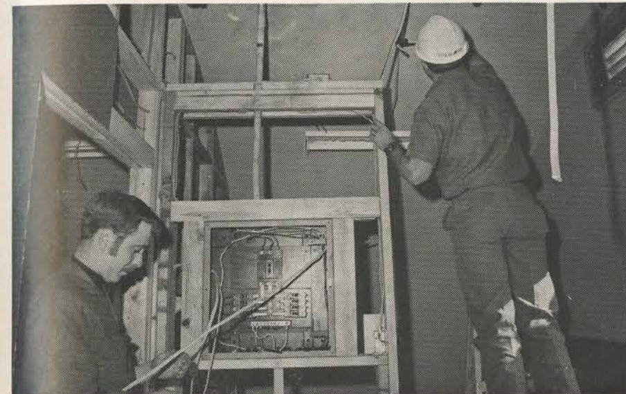
SEABEES FROM NMCB-40 INSTALL WIRING AT THE PP&K BUILDING.
