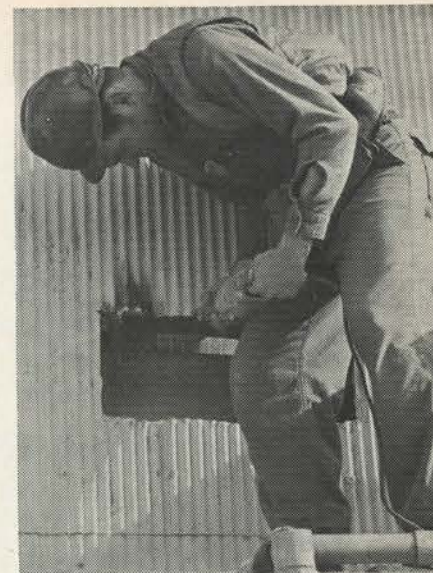
A PUBLIC WORKS SEABEE RIVETING.
