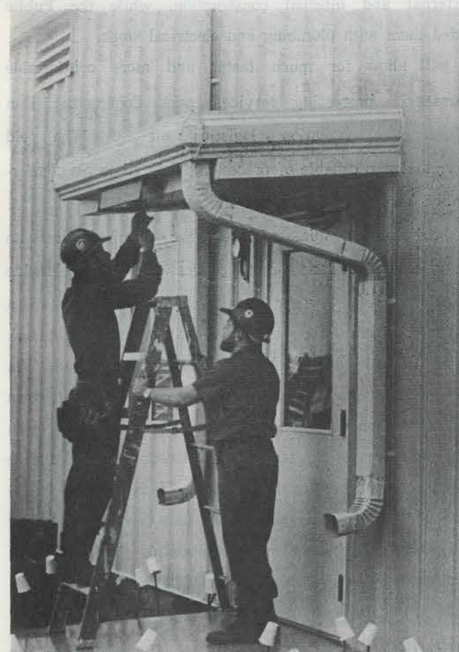
Construction Engineer Third Class George F. Letourneau (L), puts the final touches on an outside light at the Air Station's new Passenger Terminal last month. CE3 Mike D. Scott steadies the ladder.
