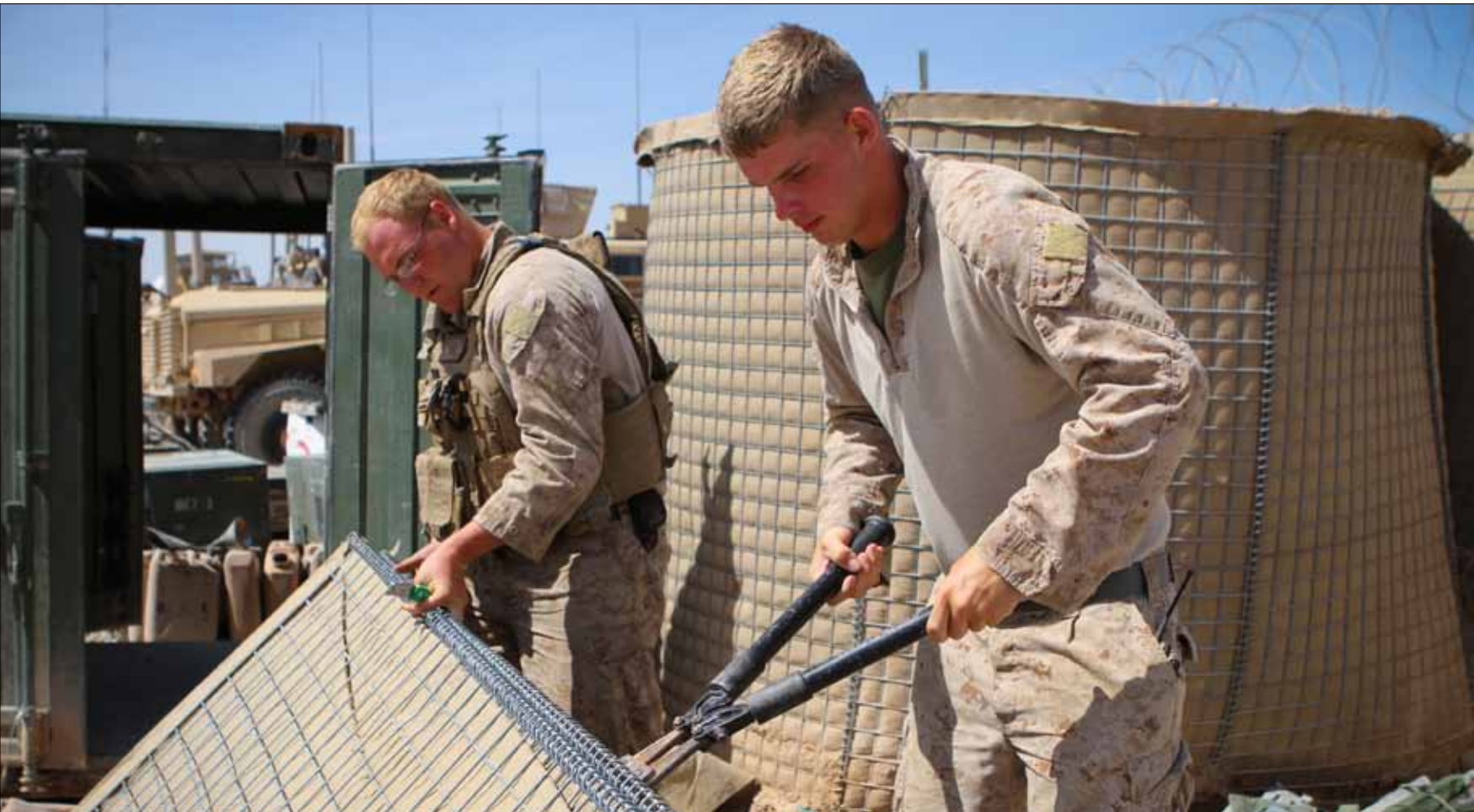
CAMP HANSON, Afghanistan — Cpl. Issac Stacy, a combat engineer serving with Engineers Platoon, 2nd Battalion, 9th Marine Regiment, cuts a HESCO wall to construct a new perimeter surrounding the base May 4, 2012. Combat engineers have torn down some of the fortified walls to shrink the base's perimeter. The Marines plan to reduce their base's guard posts in half by the end of their seven-month deployment.
