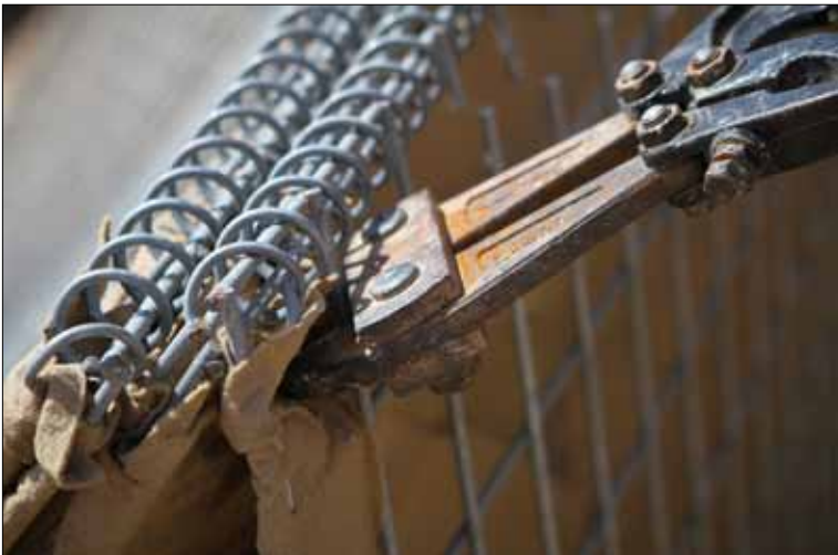
CAMP HANSON, Afghanistan — Cpl. Issac Stacy, a combat engineer serving with Engineers Platoon, 2nd Battalion, 9th Marine Regiment, cuts a HESCO wall to construct a new perimeter surrounding the base May 4, 2012. Combat engineers have torn down some of the fortified walls to shrink the base's perimeter. The Marines plan to reduce their base's guard posts in half by the end of their seven-month deployment.
