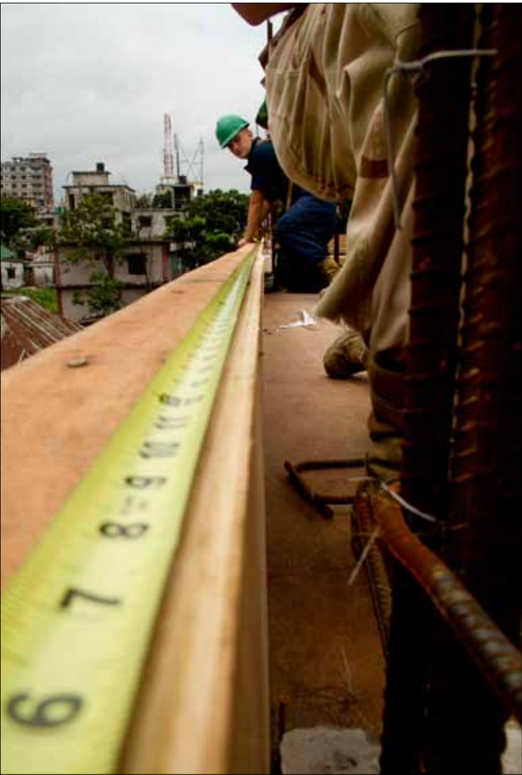
DHAKA, Bangladesh — Cpl. Tyler D. Teigen, a Marine Wing Support Squadron 171 combat engineer, measures a form before installing rebar in Dhaka, Bangladesh, Sept. 6, 2012. MWSS-171 went to Bangladesh as a part of an Engineering Civil Action Program to enhance the relationship between the United States and Bangladesh by building the second story of Hazi Joynuddin High School.
