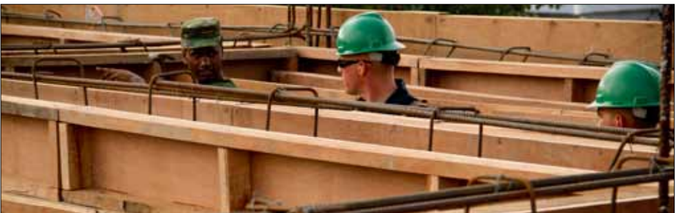
DHAKA, Bangladesh — Marines Sgt. Brian D. Davis, right, and Cpl. Kenneth R. Hornung, both Marine Wing Support Squadron 171 combat engineers, work with a Bengali soldier in Dhaka, Bangladesh to install rebar Sept. 6, 2012.
